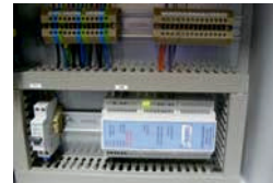
Lavero Operating Room Controller (designed and built by Prestyl USA),
