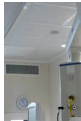
Prestyl's hospital series heaters installed
