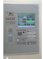
Operating room control panel
